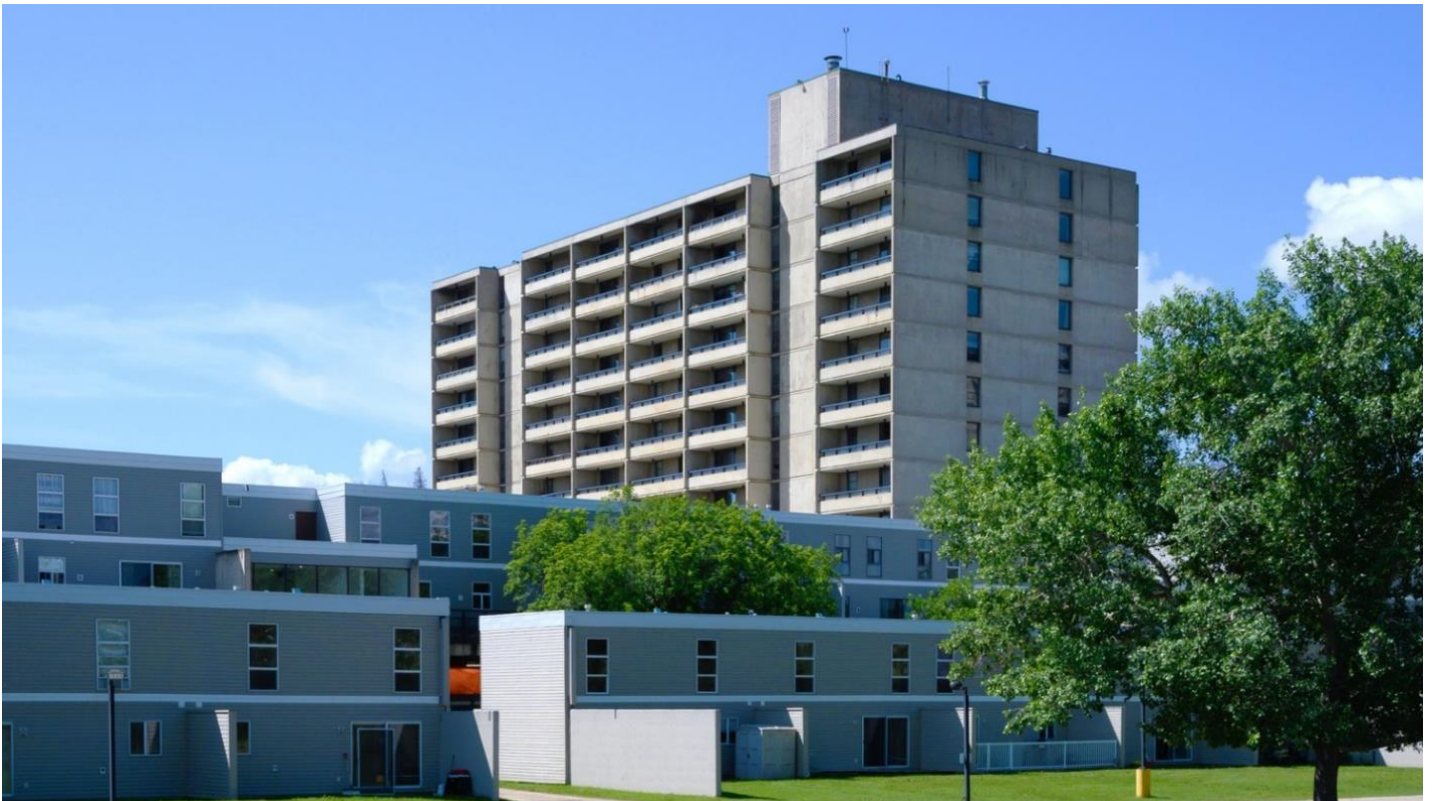
Lower Mews and Tower One
