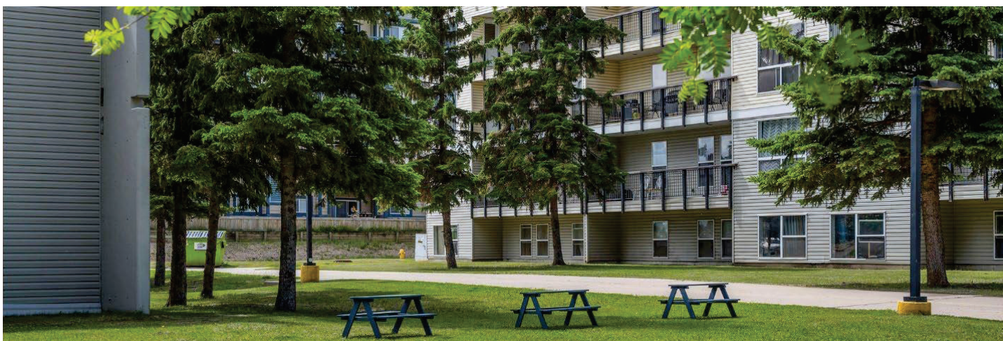
Interior Courtyard and Low Rise
